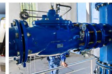
Construction of regulation and measurement manhole including electromagnetic flow meters and automatic control valves, WS Skopje (North Macedonia)
