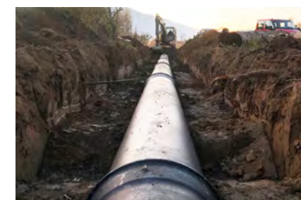
Streževo irrigation system, DN 600 and DN 800 (North Macedonia)
