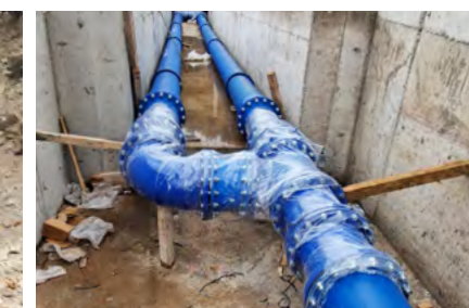
Reconstruction of the main water supply network in municipality of Stip, DN 400 (North Macedonia)
