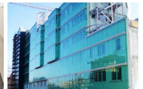
Negative pressure drainage system (EPAMS) for the Pediatric Clinic in Ljubljana (Slovenia)
