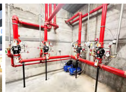
Supply and installation of sprinkler system (wet and dry type) in Belamionix Shopping Mall, Tuzla (Bosnia and Herzegovina)
