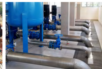
Construction of 11 pumping stations for the sewage system in Herceg Novi (Montenegro)
