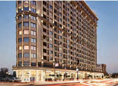
Sprinkler system and pumping station in the Adora Flatiron residential-commercial complex in Skopje (North Macedonia)
