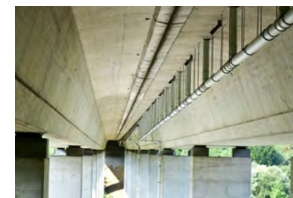
Renovation of drainage of the Lijak viaduct (Slovenia)
