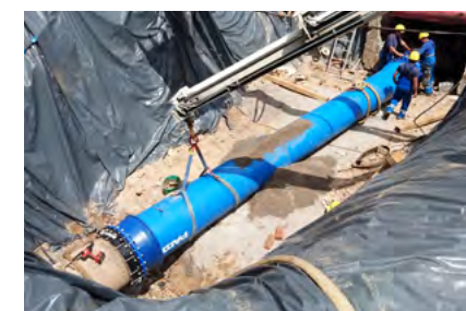
Replacement of water pipeline, DN 700, Verovškova street (Slovenia)
