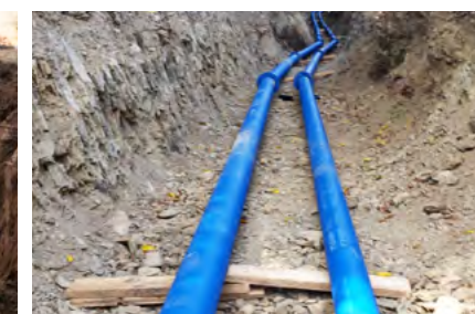
Construction of Tolminski Lom water-supply network, test pressure 63 bar (Slovenia)
