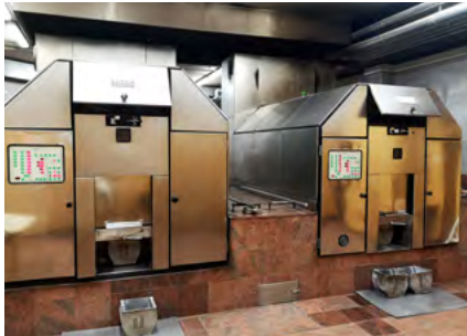
Supply and installation of the TABO-CS incinerator in Maribor (Slovenia)
