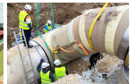
Installation of mechanical equipment and pipes, execution of electrical installations, Central wastewater treatment plant Ljubljana - phase III (Slovenia)
