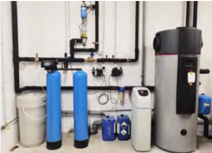
Victaulic system for distribution of technological water for heating and cooling in Precision Resource (Slovenia)
