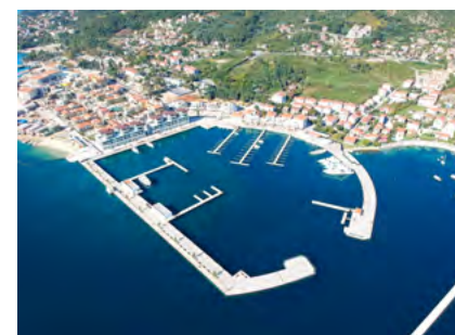
Water supply and sewage systems in the luxury Portonovi marina (Montenegro)
